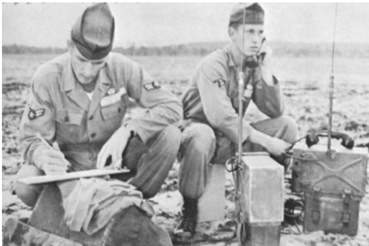
Controlling air drop from the ground. circa 1954.
